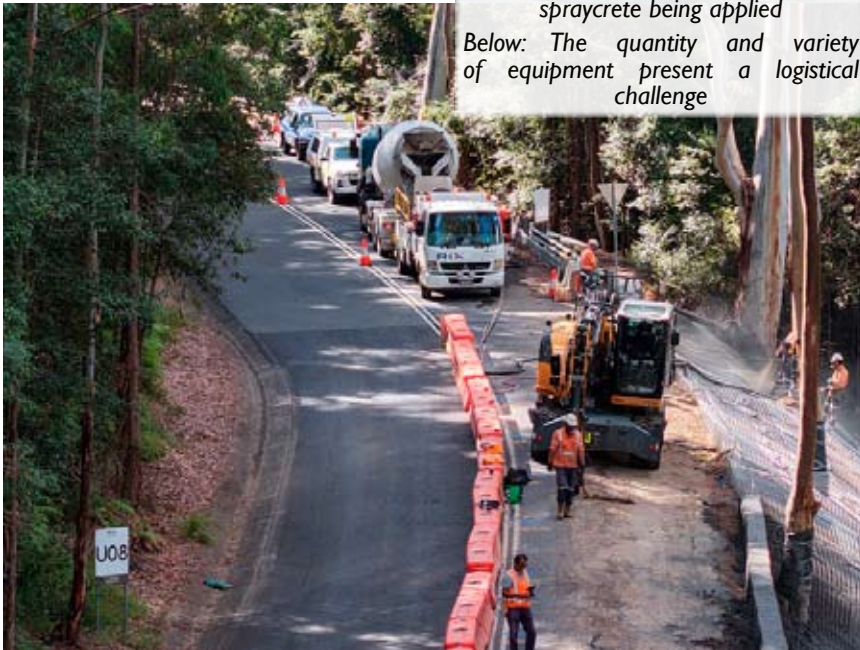
Above: Soil nails, reinforcing mesh and water drains in place with the final spraycrete being applied
