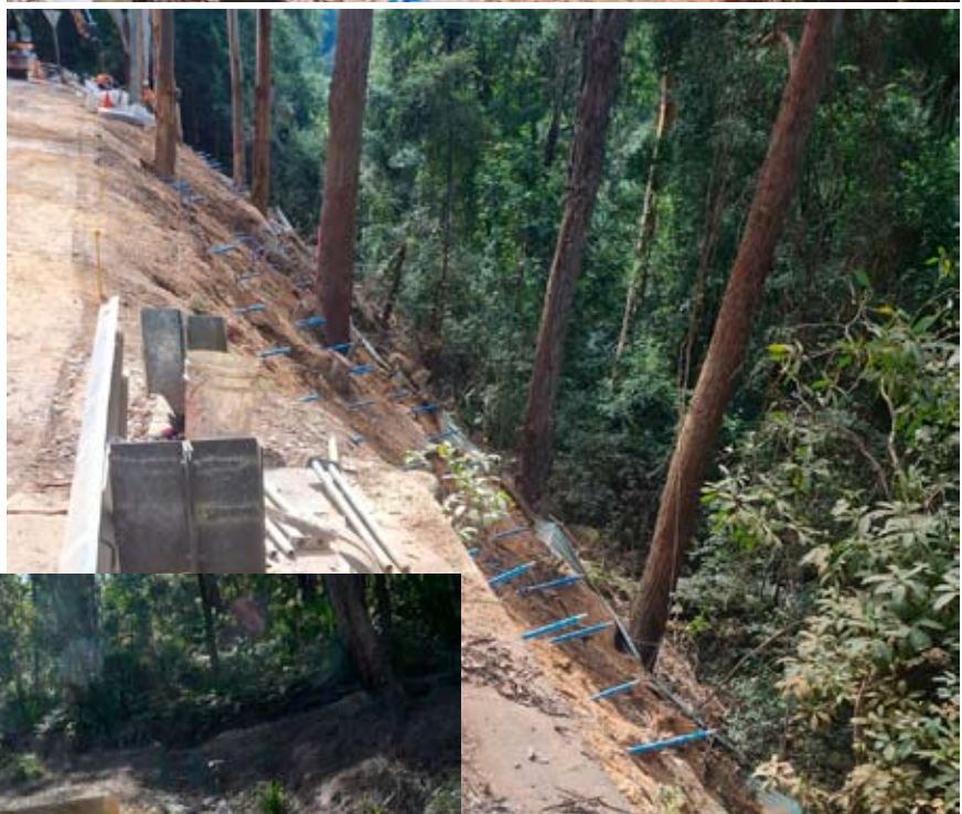
Above: Down the divvy at Greengrove - Soil nails used to stabilise the slope with reinforcing mesh & concrete to come
