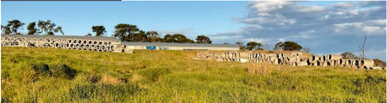
View of the pipes from Cherry Lane
