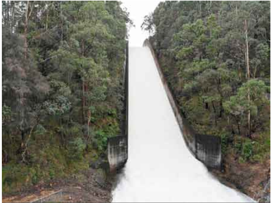
July 2022 - Mangrove Creek Dam spillway sees it's first overflow
