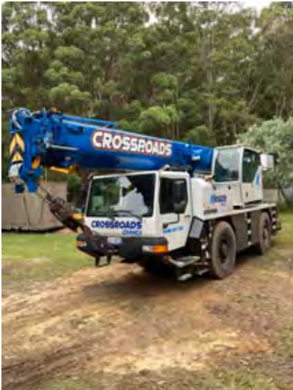
Right: Relocating a portable building to the Australia Wildlife Walkabout Park at Calga Below: 40t all-terrain crane
